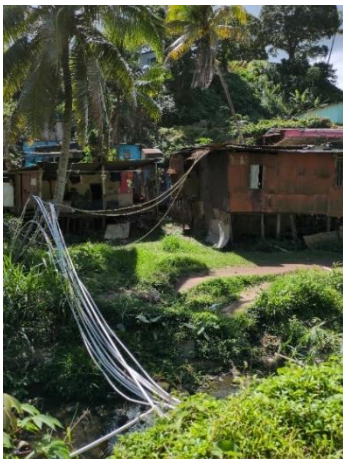
Figure 14: Settlement internal pipe networks overcoming a topographical barrier
