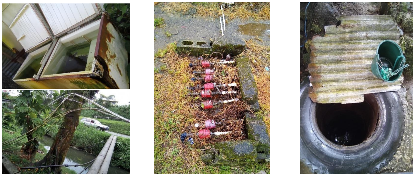
Figure 3: (a) Water stored in old fridges, Tagabe Bridge, Vanuatu (b) Water pipes after the meter in a settlement in Fiji (c) Group or “gang” meter, Efirica, Fiji (d) Shallow well in Blacksans, Vanuatu
