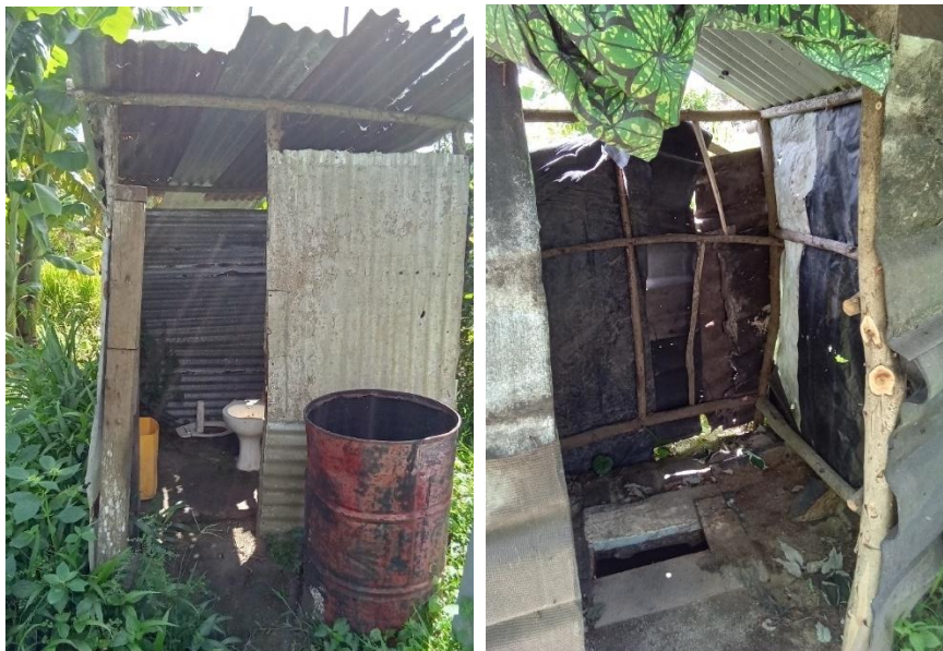
Water-based toilet (L) and dry pit latrine (R) in settlements in Port Vila, Vanuatu (Photo: USP)
