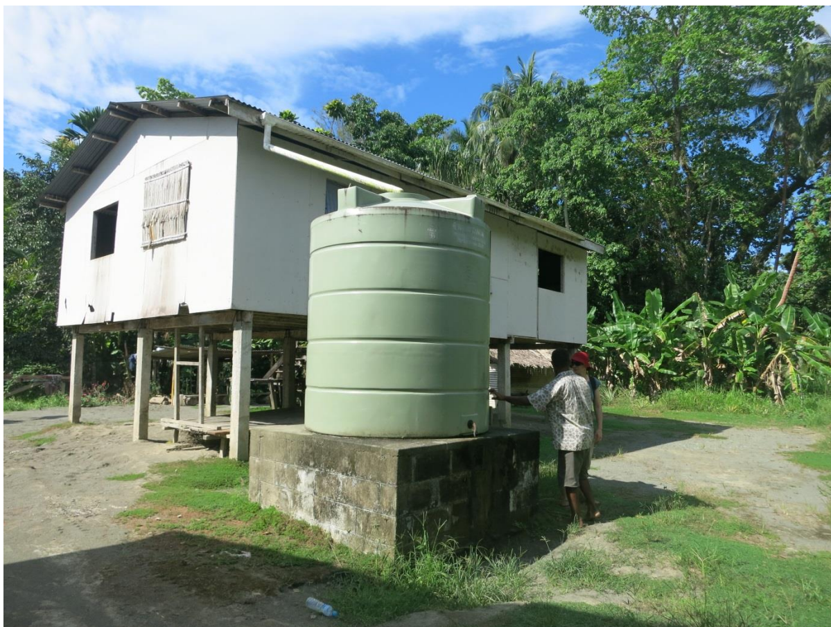
Figure 4.11. Partly functional communal rainwater tank (no tap) in Suaghi village, Guadalcanal, Solomon islands.
